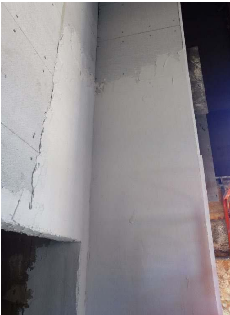
FIGURE 6: CEMENT RENDER INSTALLATION
