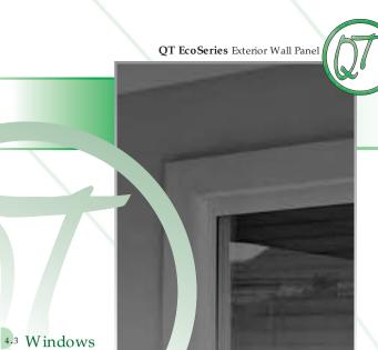
Wherever possible windows and associated flashings should be installed prior to the installation of the QT®EcoSeries Wall Panel. When ordering the window frame it is essential to plan where the window flange will be positioned either flush with the stud frame, flush with battens or even over the panel.
